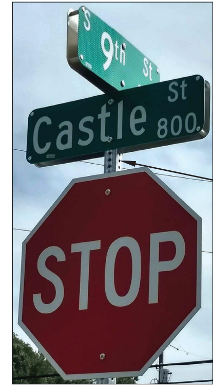
STANDARD STREET NAME SIGNS INSTALLED ABOVE A STOP SIGN (BOTTOM SIGN PARALLEL TO STOP SIGN) FIGURE 2.2
